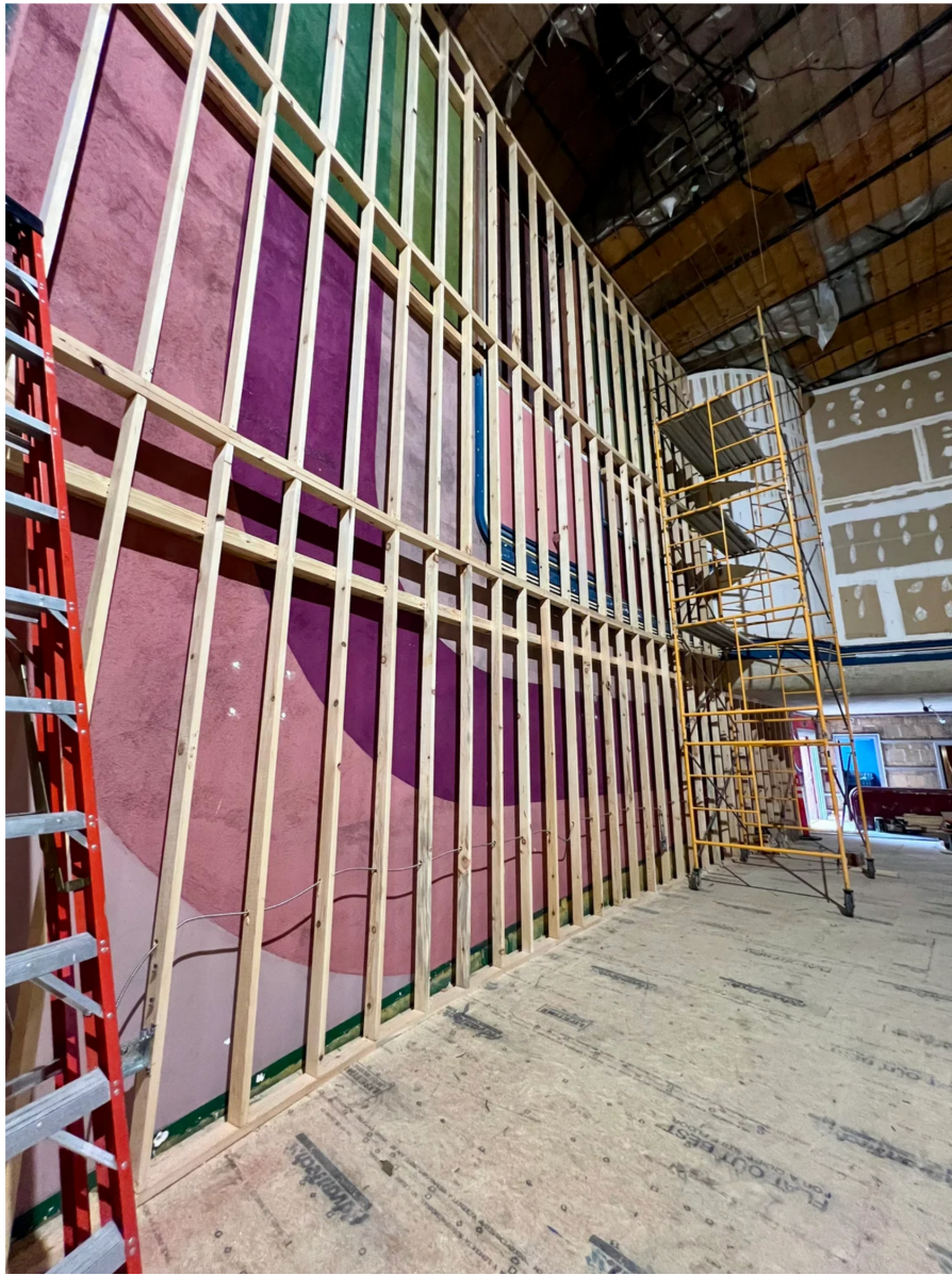
Studs on North Market Street side of the future event space.
