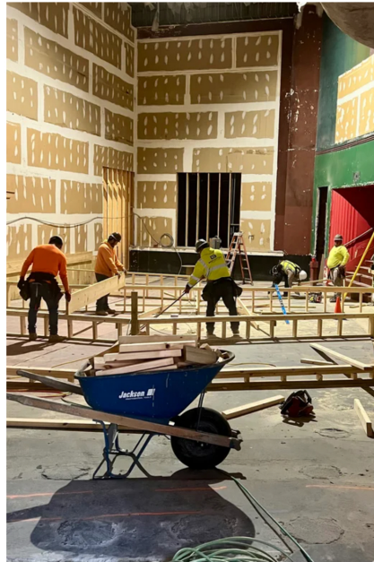
Day 2: framing the supports at 2:45PM
